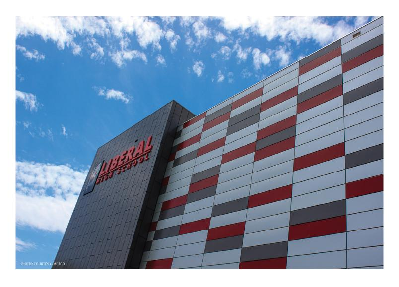
Retrofit cladding solutions, including rainscreen systems, over-roof assemblies, aesthetic wall upgrades, and engineered deck systems over pool areas, offer a practical, low-disruption path forward. These systems address not only energy inefficiency and weather protection but also allow schools to renovate problematic spaces and rejuvenate tired exteriors.
